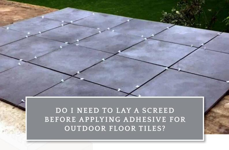
Ideally, yes. Laying a sturdy screed will provide the best possible foundation on to which your tiles can be fixed and will prevent flexing and slippage. It's especially important to have a fully cured (we advise leaving a concrete screed to cure for at least 6 weeks prior to applying an adhesive bed) if you're installing 20cm thick porcelain slab tiles as these heavier, sturdy tiles require a thick bed of around 20mm to ensure the tiles fix properly.
