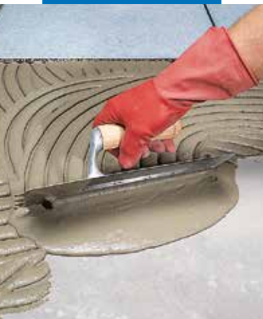
Spreading with semicircular notched trowel
