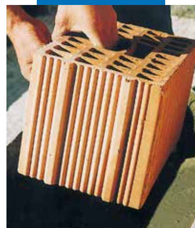
Dipping a concrete block in Adesilex P4
