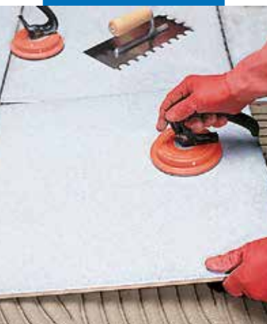
Laying large size tiles
