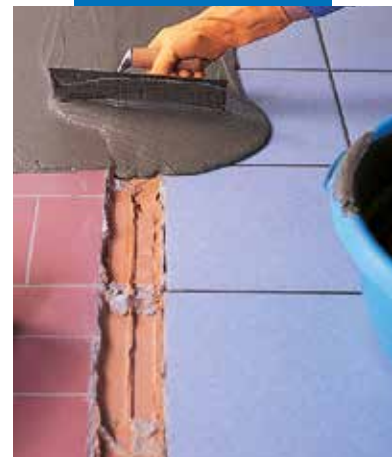
Smoothing existing flooring with Adesilex P4
