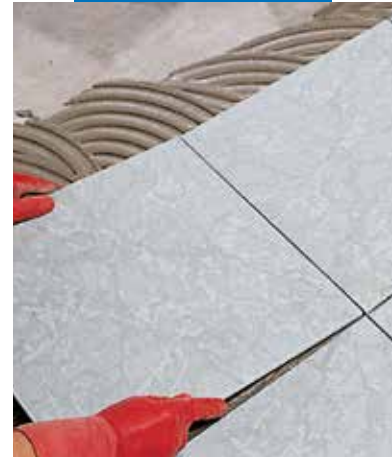
Laying porcelain tiles
