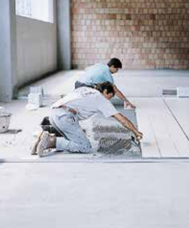
Laying porcelain tiles in a factory
