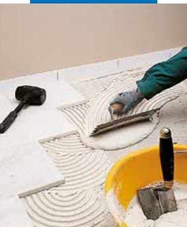
Laying white Carrara marble with Granirapid white
