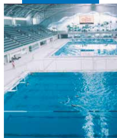
An example of an installation of mosaic and klinker in a swimming pool - Olympic Centre - Sydney (Australia)
