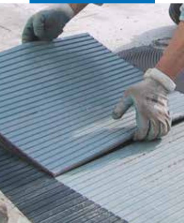
Laying vitreous mosaic with Granirapid white
