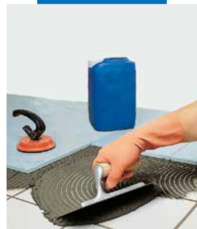
Laying agglomerate tiles over existing ceramic tiles with Granirapid grey
