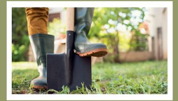
Dig out the area to be tiled making sure it is stable and to an approximate depth of 200mm.
