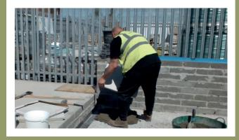
Lay the previously primed tiles into a solid bed of Rock Tite Mortar approximately 25 - 80mm thick.
