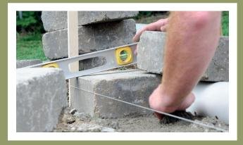
Set out the area to be tiled using a horizontal level line and a second sloped line to create a fall, as set out below.
