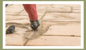
Compact the joints and finish them with a jointing tool, if voids appear refill and re-finish. Brush off any excess grout.
