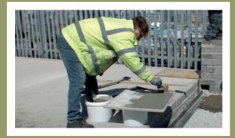
Apply Rock Tite Porcelain Primer to the back of the tiles and allow to dry. Brush or roller are the best methods of application.
