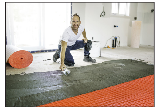
Mix and lay adhesive with notched trowel
