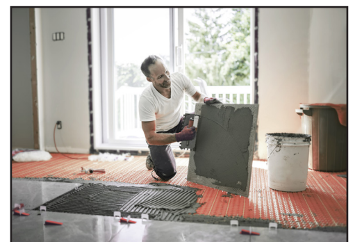
Install tiles onto membrane
