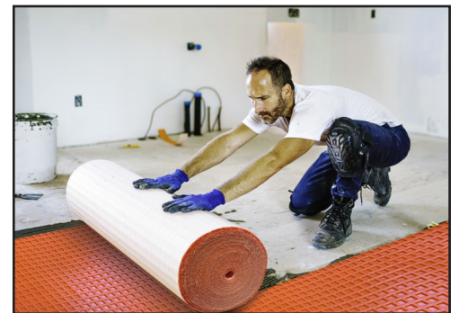
Position and install membrane
