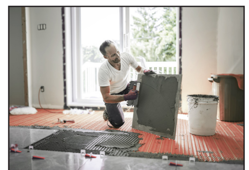
Install tiles onto membrane
